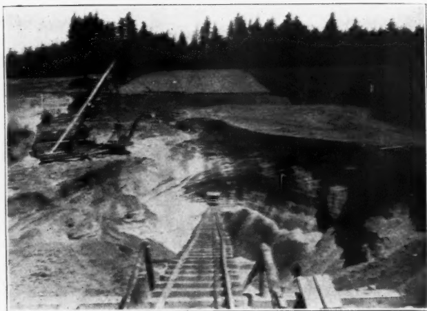
Looking Down Trestle Into Pit
